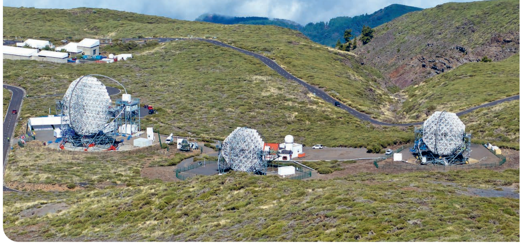
Figure 12: Visible in the photograph, from left to right: the first Large-Size Telescope (LST1) of CTA (24 m mirror-diameter), FACT (4 m) and the MAGIC telescopes (17 m) at Los Roches de Muchachos, La Palma. The LST1 was inaugurated in October 2019 (Image: CTA Collaboration)
